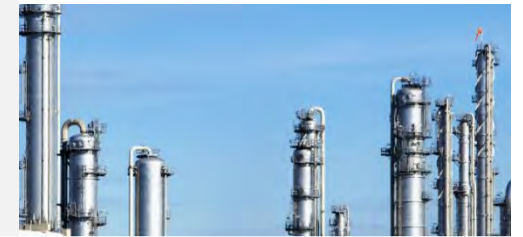
Petrochemical & Refinery process
